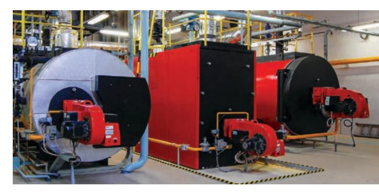
In general, the main task of the burner is to create heating, which is selected according to the need, the desired burner. Burners are used to convert water to steam, heat heat transfer fluids, direct heating in cooking and oxidizing, provide heat to dry products, and other special uses. One of the biggest uses of the burner in the heating industry is as a combustion engine for boilers. Different types of boilers use burners with different working capacities.
