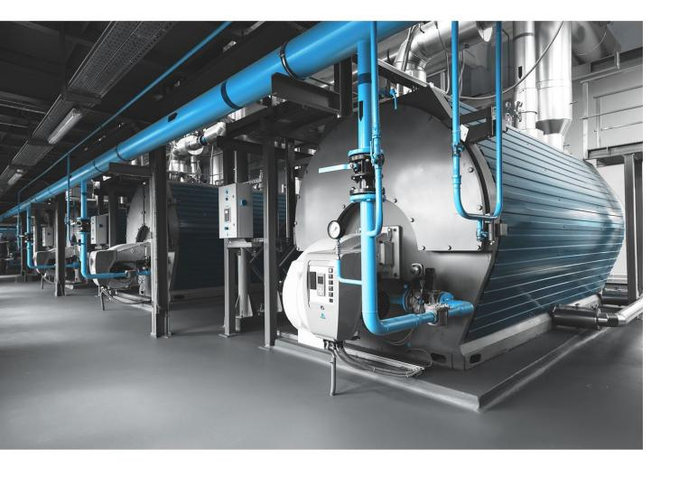
An industrial boiler is essentially a giant industrial kettle used for heating water or other fluids to high temperatures. This hot fluid serves various purposes within a facility, such as generating steam to power turbines for electricity production, supplying heat for large-scale industrial processes (drying products, sterilizing equipment), or providing hot water for building heating systems.
