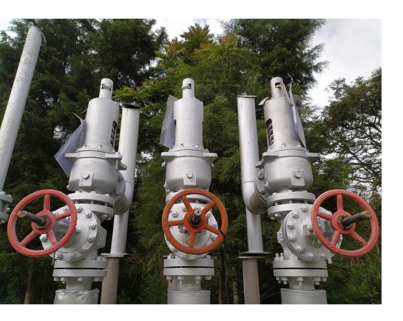
A safety valve is a pressure release mechanism that acts as a fail-safe for pressurized systems like boilers or pipelines. It essentially functions like a pressure relief valve on a pressure cooker. By automatically opening when pressure builds up beyond a safe limit, it safeguards against catastrophic events like explosions or ruptures. Imagine it as a built-in emergency hatch that vents excess pressure to keep the system from bursting.
