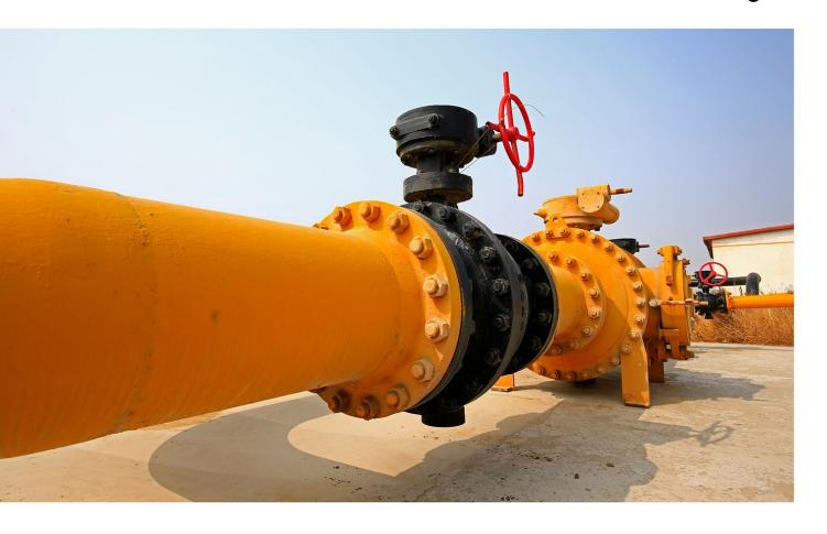
A flanged valve is a type of valve that utilizes flanges on either end to connect to pipes or other equipment. These flanges are bolted together with a gasket in between, creating a secure and leak-proof seal. Flanged valves are ideal for high-pressure applications because of their strong and reliable connection. They are also easy to install and remove, making them a popular choice for industrial processes, power plants, and water treatment facilities.
