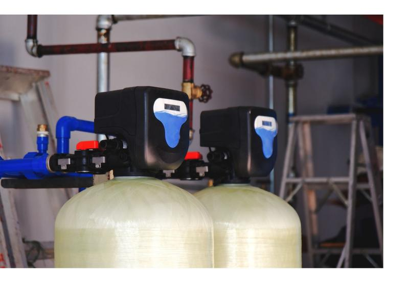
Industrial water softeners tackle a common problem – hard water. They act like filters, removing dissolved minerals like calcium and magnesium that cause scaling and contribute to inefficiencies in boilers, cooling towers, and other equipment. This softened water improves overall performance, reduces maintenance needs, and extends the lifespan of equipment in industrial facilities.
